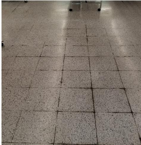
Subsequent MVER tests, which were completed in Spring, 4 years after the initial tests, were 7.2 lbs or less (range of 3.2-7.2 lbs) with a maximum RH of 94% (range of 90-94% RH) and pH readings ranging from 8.4-9.4. Changes in environmental conditions were such that the adhesive could not protect the flooring from MVER.
