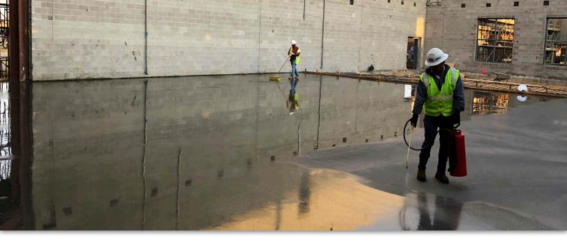
The CS2000™ system is applied the day of the concrete pour or as soon as weather conditions permit, prior to any other chemical treatment. Construction traffic can resume as early as 2-4 hours after the CS2000™ application.
